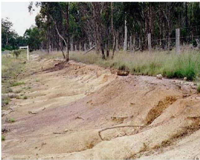
Plate 10 Incipient erosion along a roadside. Areas like this should be targeted for roadwork maintenance to overcome erosion and to stabilize the site ready for revegetation
