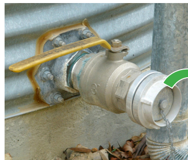
Figure 6 Ball Valve 65mm Storz fitting
